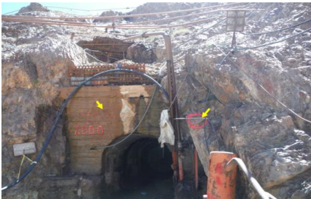
Figure 49: Anchor points at the entrance of the 2000 level
