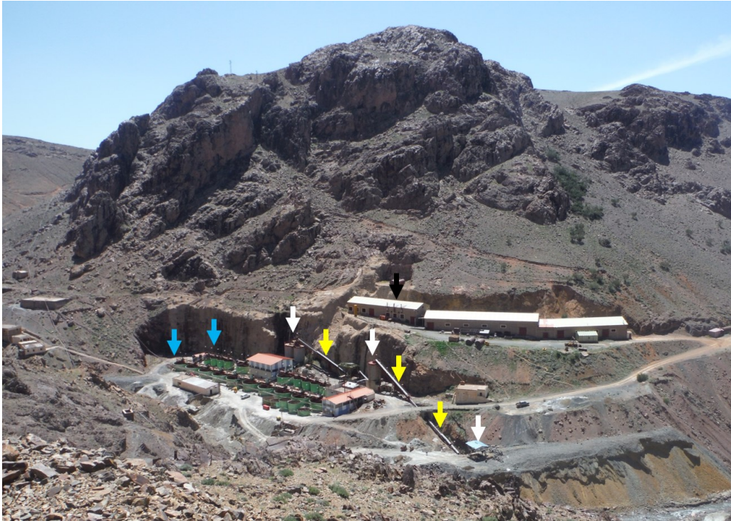
Figure 13: A general view looking west of the Zgounder mill installations showing the conveyor (yellow arrows), storage bins with crushers (white arrows), two cyanidation lines with counter-current decantation (blue arrows) and diesel generators (black arrow)
