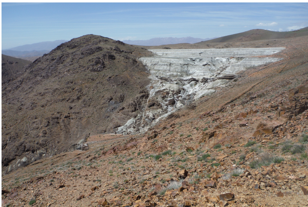
Figure 27: Tailing behind the old dam
