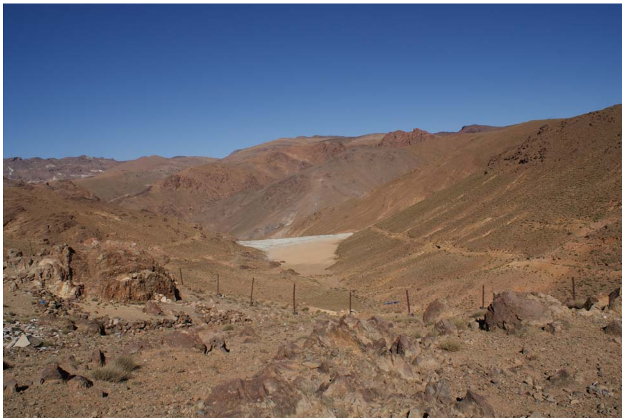
Figure 29: Northeast view of the recent tailings dam.
