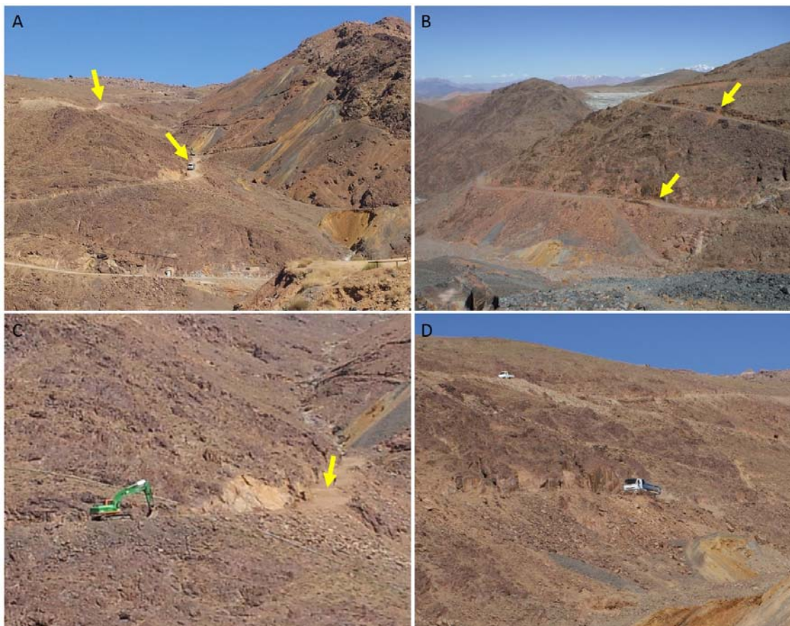
Figure 10: Broadening the gravel trail from level 2000 to 2175 at Zgounder silver mine.
