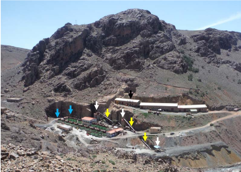
Figure 13: A general view looking west of the Zgounder mill installations showing the conveyor belts (yellow arrows), storage bins with crushers (white arrows), two cyanidation lines with counter-current decantation (blue arrows) and diesel generators (black arrow).
