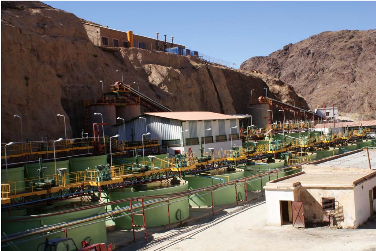
Figure 15: View of the cyanide leaching tanks & counter-current decantation thickeners.
